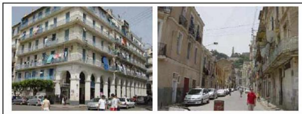
(1) Houses and shops Masonry buildings
