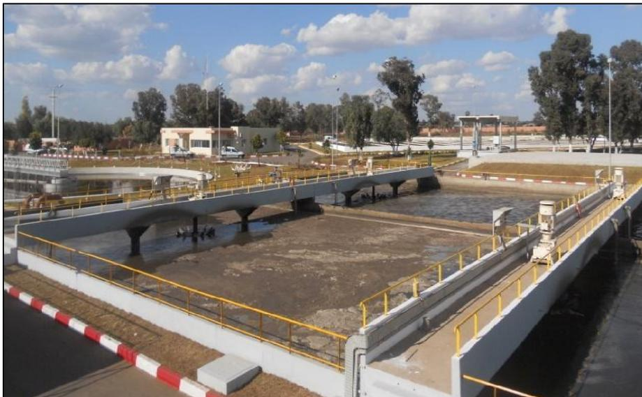
**Figure 4:** Photo of the biological basin of the treatment plant in the city of Khouribga.
