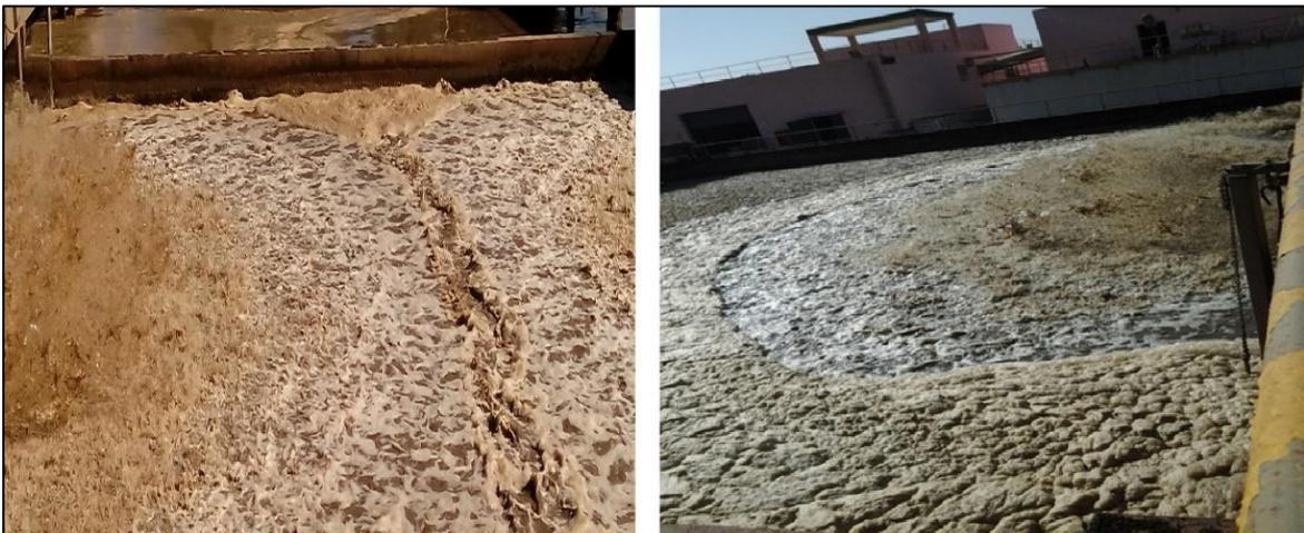
**Figure 18:** Biological foam on the surface of the aeration basin in WWTP.
