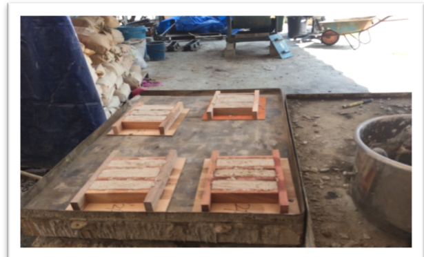
Figure 6: Compacting the mortars on the vibrating table
