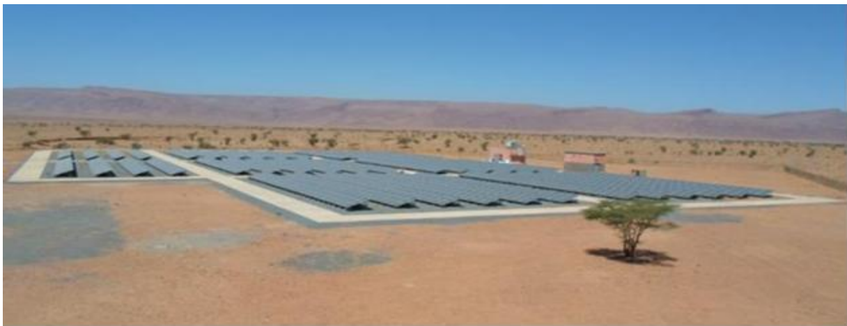
Figure 1: View of the 806.52 kWp grid-connected PV system installed at the Assa Town, southern Morocco.
