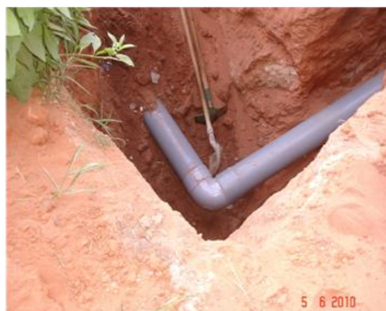
Figure 3: The elbow to the laying of the siphon.
