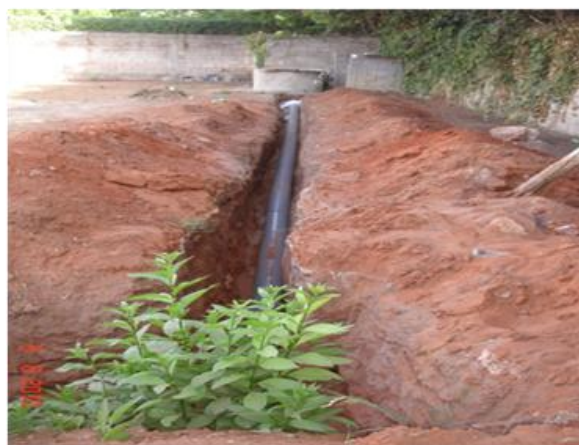
Figure 2: The trench and pipe lying.
