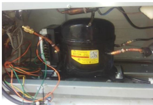
Figure 2: Installation of DC compressor
